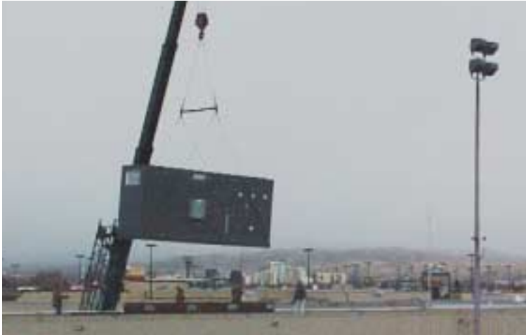
▲ TMP-15000 unit being hoisted onto rooftop
