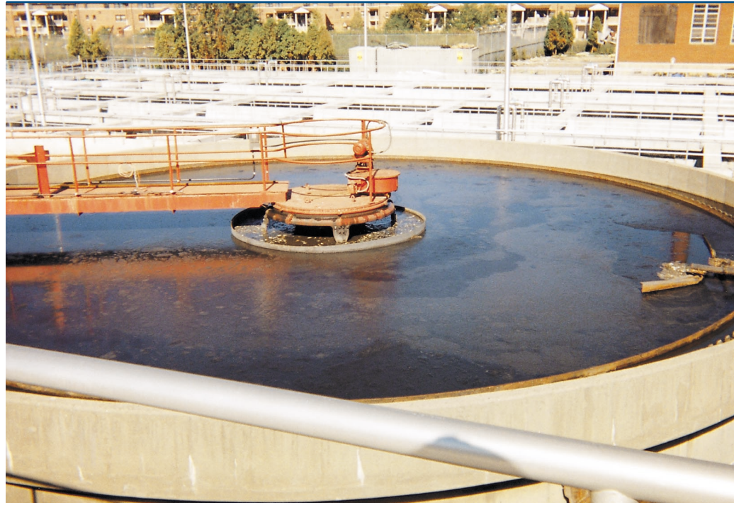
▲ Wastewater Sludge Settling Tank
